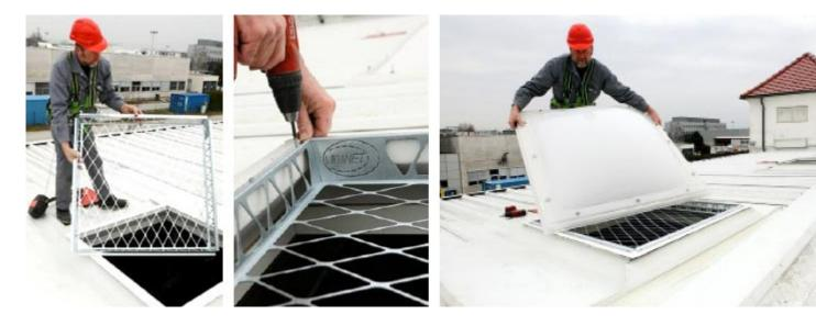
Can be fixed on virtually all intact upstands. Likunet® is inserted in the upstand and fixed with the screws provided. The grid can be cut out in small areas for fan motors. For smoke and heat extraction bridge structures, using a domed rooflight with integrated net between the walls is recommended.
