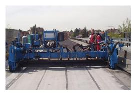
for the automatically installation of mastic asphalt used in road building and hall construction
